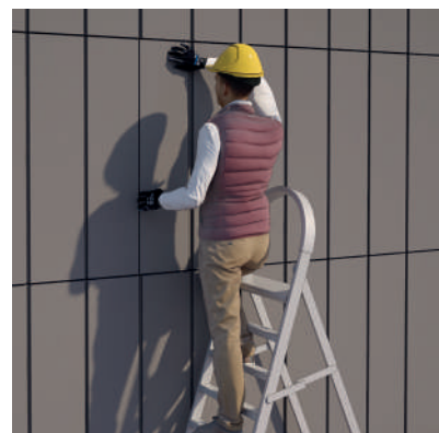
Check the alignment of the installed product and the stability.
