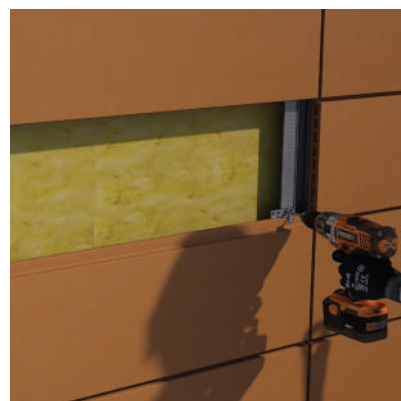
Install the high clip PITA02.
