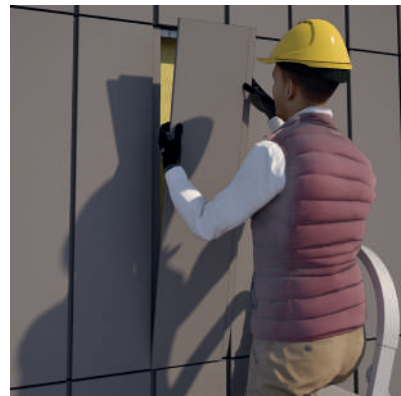
Install the V-clip® on the lower part of the replacement terracotta product. Place the terracotta product by clipping the V-clips® on the bottom rail.
